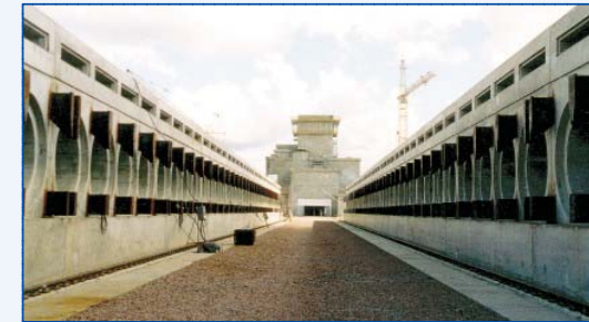
Spent Nuclear Fuel Storage at Chernobyl NPP for RBMK fuel
