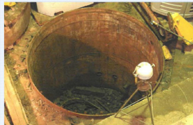
Emptied reactor shaft
