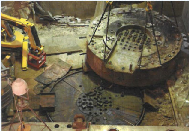
Dismantling of reactor head
