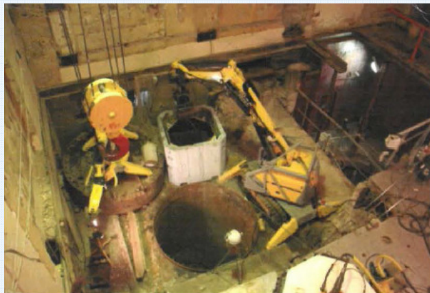
After dismantling of reactor internals
