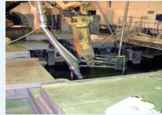
Channels cutting in the reactor pool
