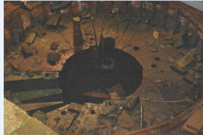
Graphite stack of reactor RFT
