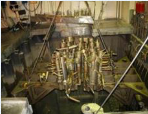
Removal of reactor internals
